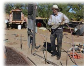
Ray drilled 5' deep holes to anchor our new carport.
